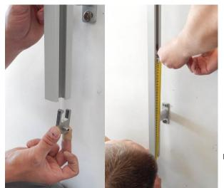
1. Insert the intermediate bar into the arm cutouts and insert the whole into the guide rails.
