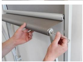
3. Make one turn of the bottom bar to roll the fabric and screw the movable part of the arm to the sides of the bottom bar.
