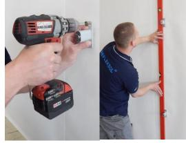
2. Drill holes, then mount the bracket using appropriate fixing system.
