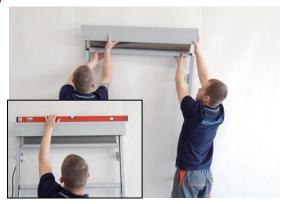
1. Put cassette on the guide rails, remembering that it has to be levelled horizontally.
