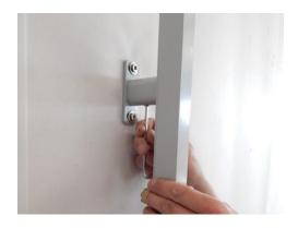
6. Loosen clamping screws, then pull out bracket bolts.
