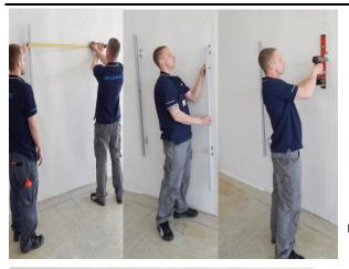
9. Use measure tape and spirit level to transfer installation places for second guide rail.
